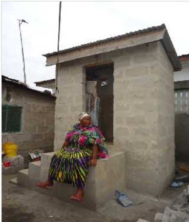
Above photo: the collapsed toilet at Zaituni’s house and Zaituni sitting in front of her new toilet
